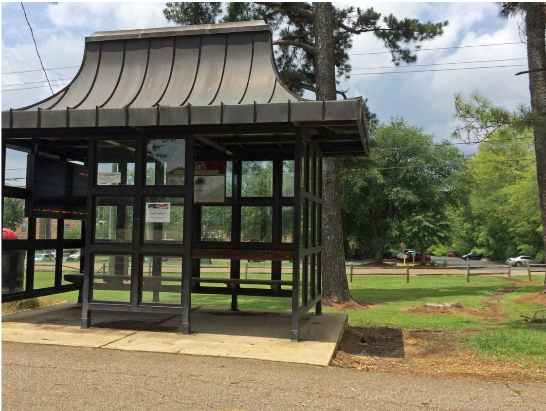
Figure 4. Starkville Bus Stop. A stop located along the Starkville-MSU Area Rapid Transit (S.M.A.R.T.). Footpaths leading toward student apartments can be seen on the far right (photo by author).
